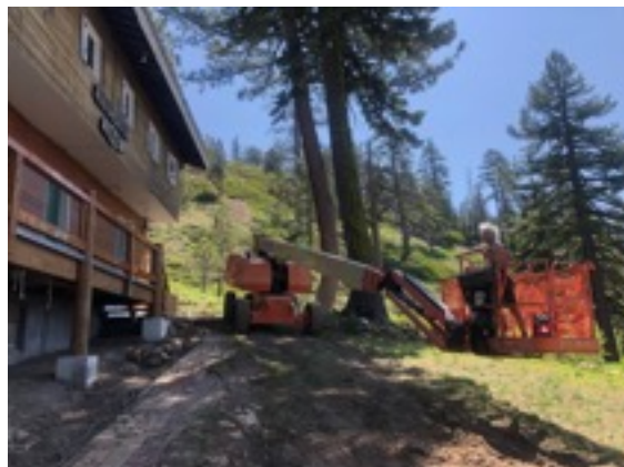
High reach crane for preparing walls
